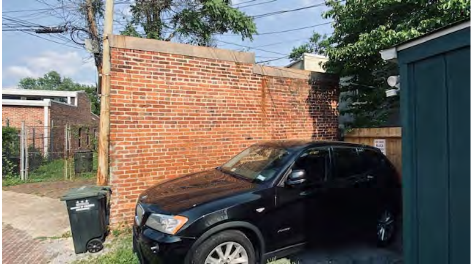
Side View from Adjacent Parking Pad
